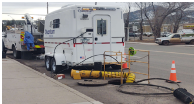
Century Link in Williams installing the fiber link from Phoenix
